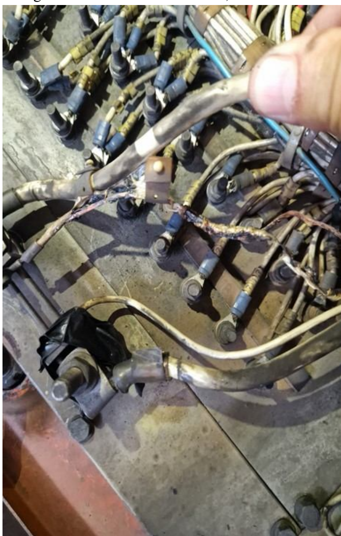
Fig. 4.15. Burnt conductor 873
