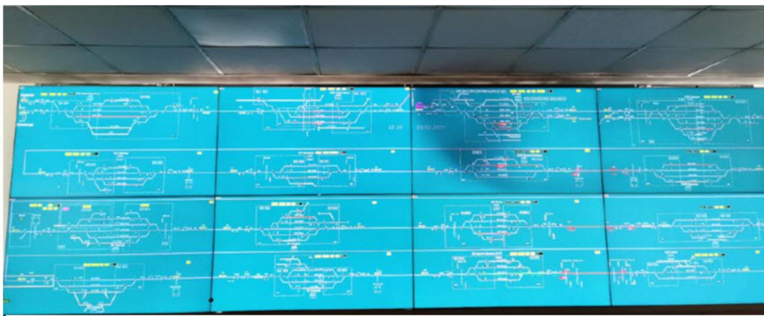
Fig. 3.6. Dispatching interlocking along the section Iliyantsi-Karlovo type TRIS CTC.
